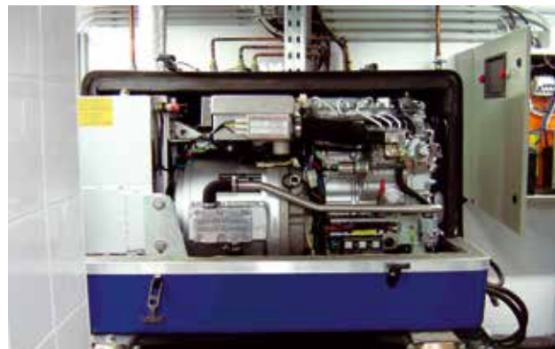
This three-phase Panda is installed in the basement. Main fuses, panel, and radiator control are fitted in electrical cabinet. Image: Kratos Kft. Hungary.
