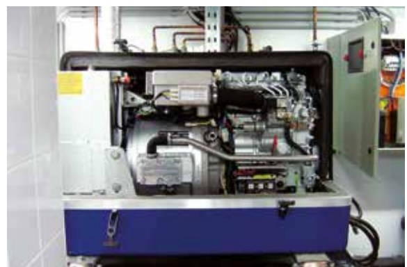
This three-phase Panda is installed in a basement. Main fuses, panel and radiator control are fitted in an electrical cabinet.
