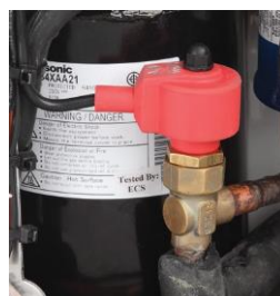
Electronic expansion valve for precise control of superheat.
